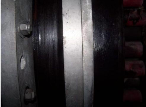
Picture 19 – Side view of floating tubesheet
