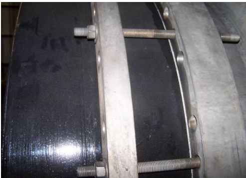
Picture 17 – No leaks in tubesheet upon testing.
